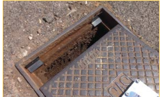
Shims positioning between cover and frame.
